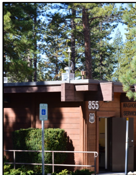
Figure 9 Incline Monitoring Site
