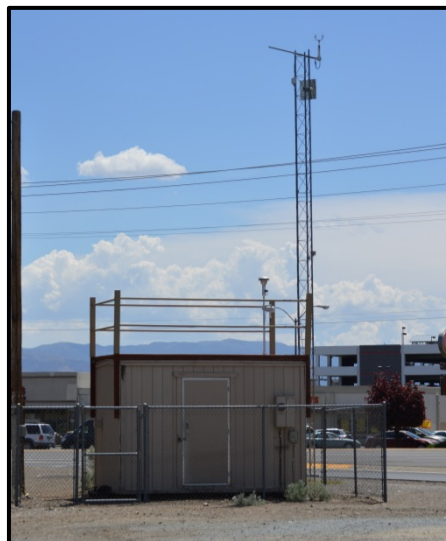
Figure 7 Plumb-Kit Monitoring Site
