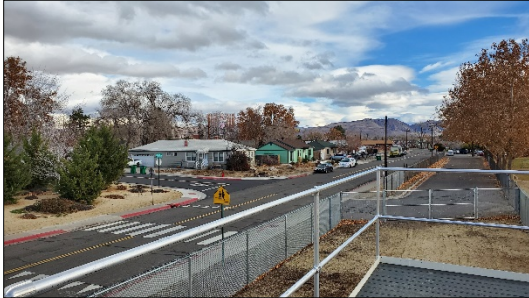
Figure 8 Looking East from the Probe
