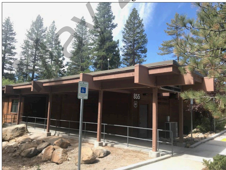
Figure 4 Incline Monitoring Station
