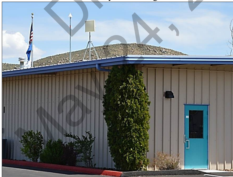
Figure 6 Lemmon Valley Monitoring Station
